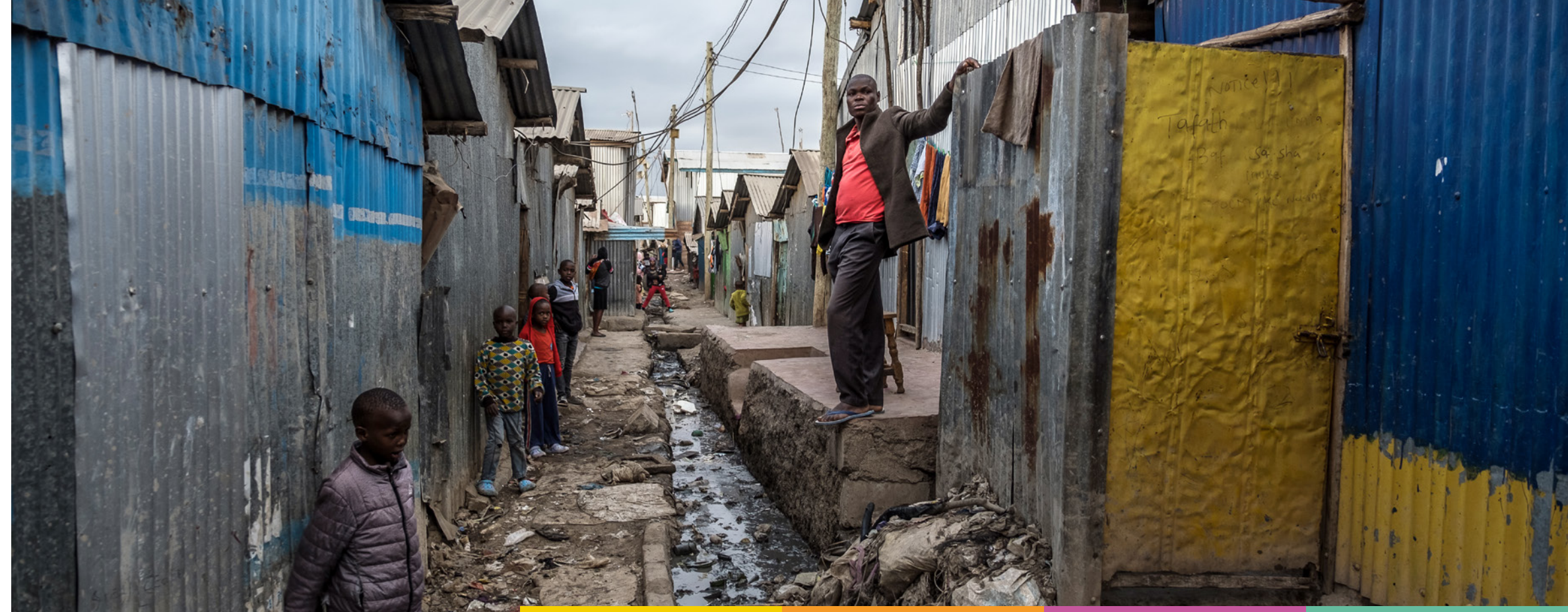
Image: People walk past open sewers in the Mukuru neighbourhood of Nairobi. A lack of proper sanitation is very common in unplanned, low-income neighbourhoods like Mukuru, and makes life unpleasant and unhealthy for residents. In 2023, working with the municipal authorities and the community, and with funding from The One Foundation, WSUP provided new pre-paid water dispensers and new connections to the main sewerage line, through a simplified sewer system (see later article). Credit: Brian Otieno, Kenya, August 2023
