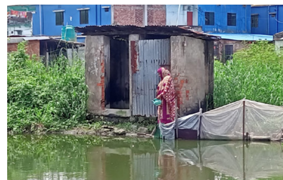
Image: Sajeda Begum stands outside the only toilet available for her and 30 families until WSUP intervened. This toilet was unlit, and frequently flooded with human waste and snakes. Bangladesh, 2021. Credit: WSUP
