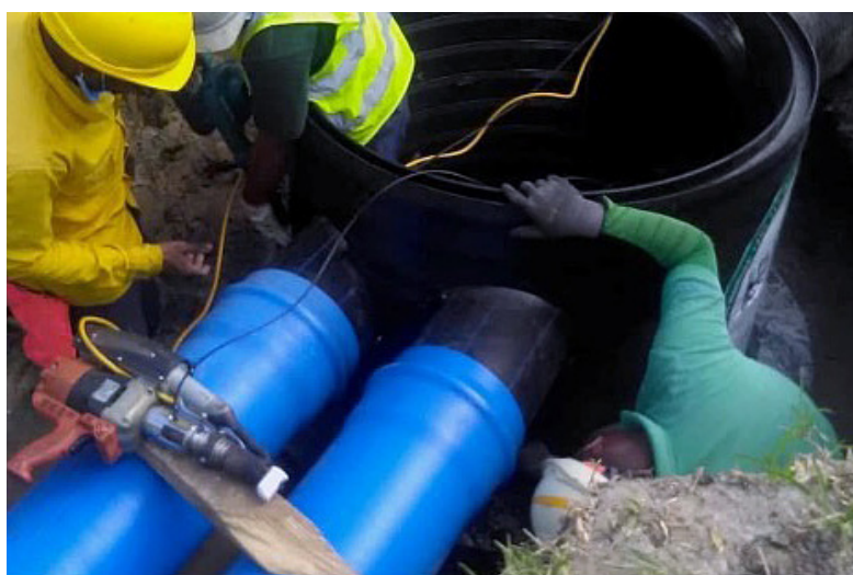
Image: HDPE Inspection chamber installation for SSS.
