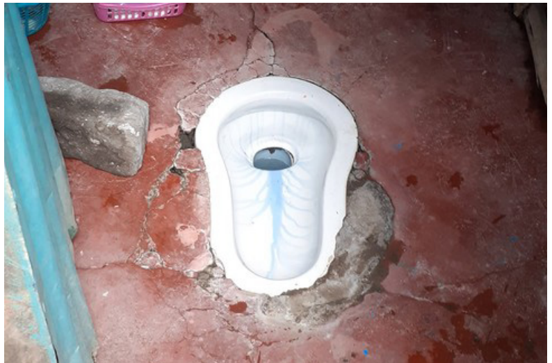
Image: Upgrading pit latrines to pour-flush toilets connected to the simplified sewer system, Mukuru, Nairobi.
