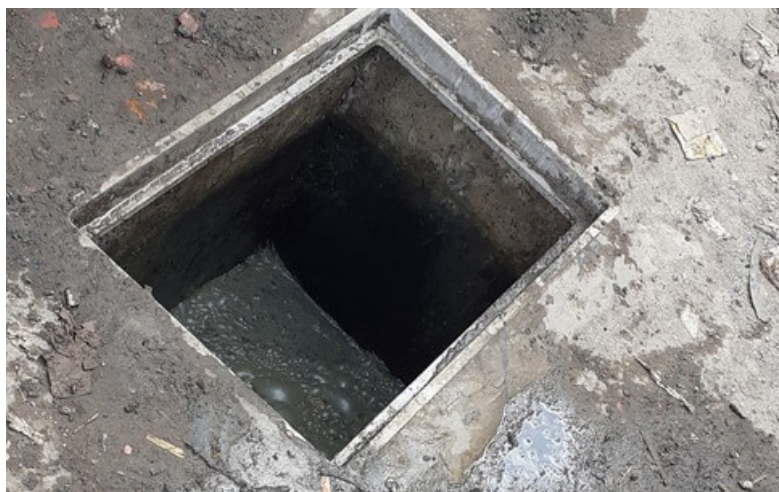
Image: Upgrading pit latrines to pour-flush toilets connected to the simplified sewer system, Mukuru, Nairobi.
