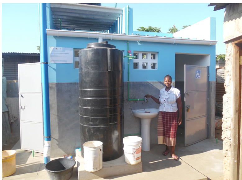
Image: Resident uses a communal washblock in Maputo, Mozambique. Credit: WSUP
