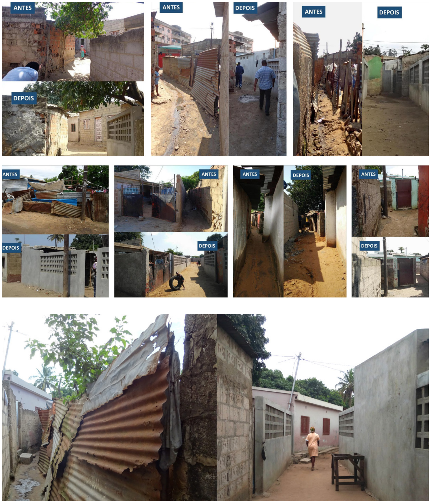
Figure 5. Typical before-after images under the Habitat Project which have created a common language between community, politicians and technicians.
