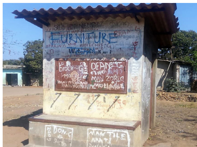
Image: A disused water kiosk in Livingstone, Zambia, built before the water utility built a new water network for the community
