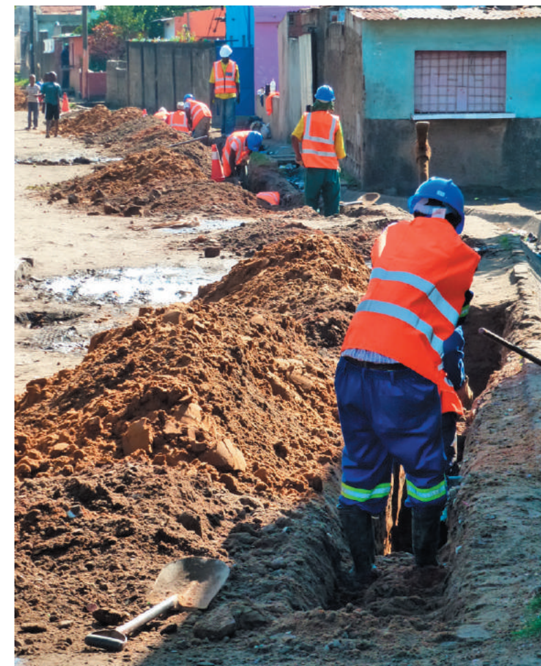
Image: Tertiary network construction in Charmanculo, Mozambique.
