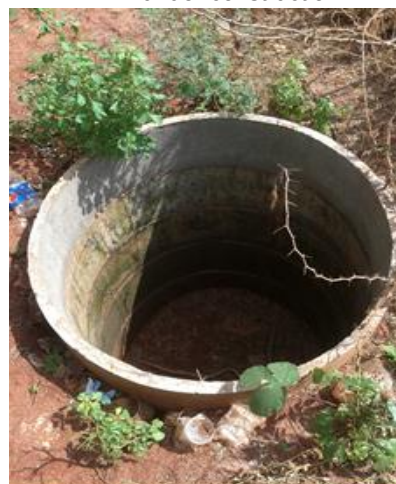
Concrete rings for pit
