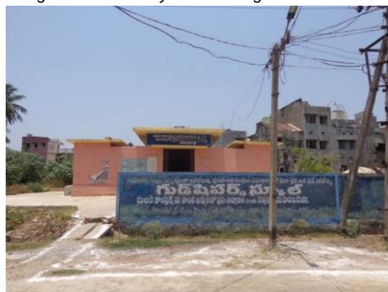
Image 9 Community toilet along the road
