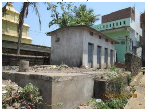
Image 6 Closed community toilet building in Zone 8 (Bheemunipatnam)
