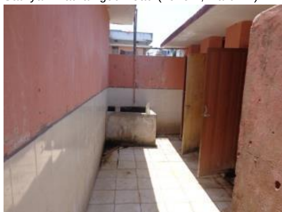
Image 24 Good Day lighting in community toilet, Sathyammathali gudi road (zone 7, ward 21)
