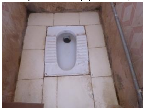
Image 29 A toilet in a pay & use facility
