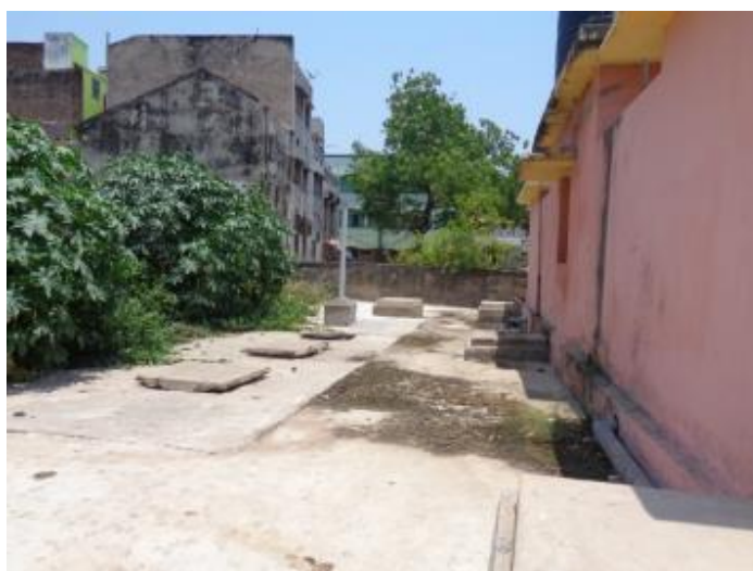
Image 19 Septic tanks in community toilet near Nookambhika temple (zone 7, ward 21)
