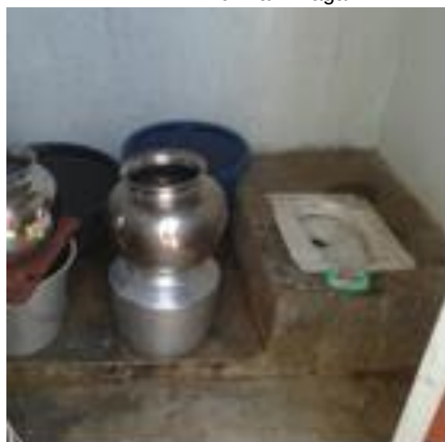
Functional toilet facility
