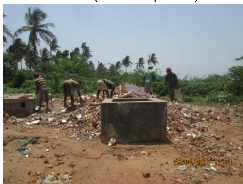
Image 7 Under construction toilet building in Zone 8 (Bheemunipatnam)
