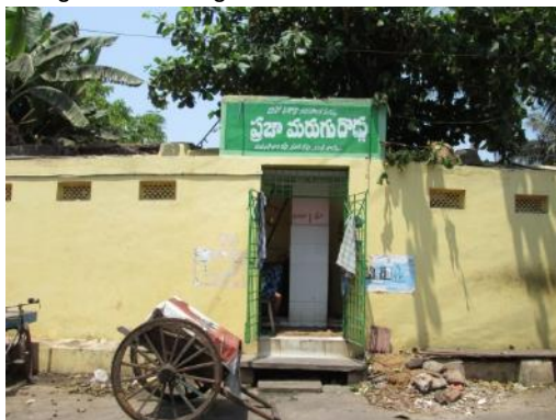
Image 12 Garbage littered in front of PT/CT
