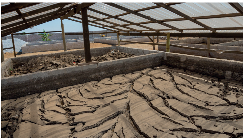
Image: Drying beds for treatment of sludge collected by the FSM service, Lusaka. Credit: Gareth Bentley
