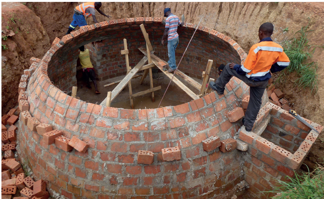
Image: FSM transfer station under construction in Chazanga, Lusaka. Credit: WSUP
