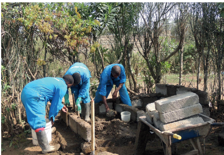
Image: Upgrading latrines in Kenya. Credit: Wanjiku Njenga
