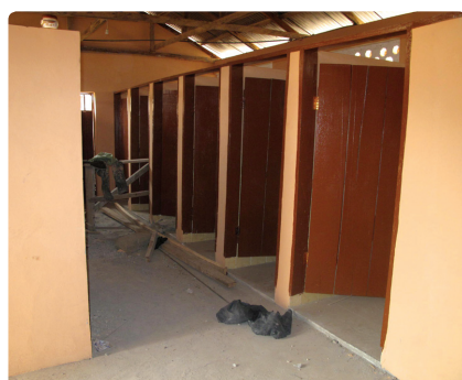
Sanitation block under construction
