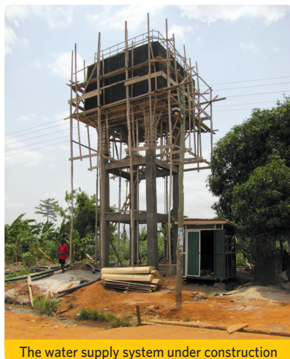
The water supply system under construction
