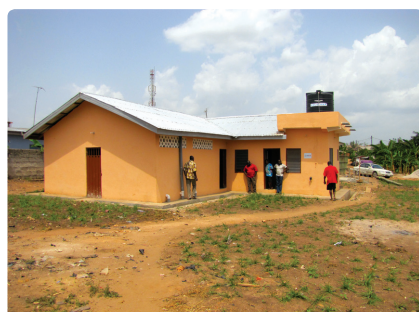
Sanitation block under construction
