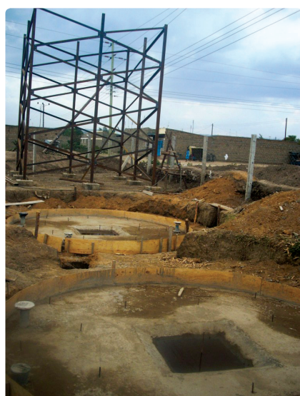
Water tank construction, Karagita
