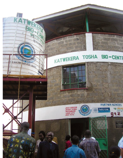
BioCentre facility in Kibera
