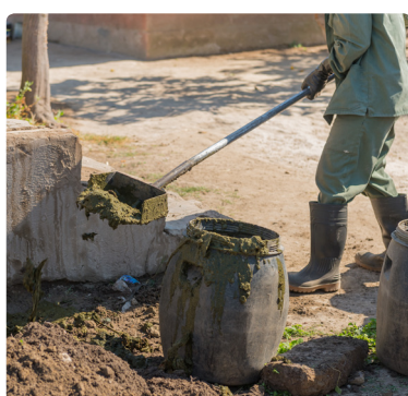
Manual emptying of a pit latrine using modified garden tools
