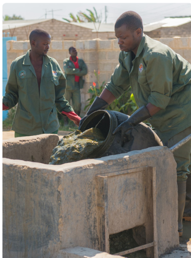
Disposal of sludge at the decentralised transfer station
